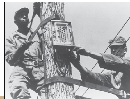
These student repairmen install a terminal box atop a telephone pole. This is an example of the practical training received in the Air Training Command installer repairman phase of the fixed wire communications course at F.E. Warren AFB. (U.S. Air Force photo)
