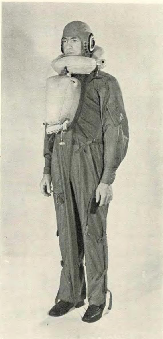
new-type suit would provide adequate buoyancy and freedom of motion for aircrewmembers in the event of bail out.
