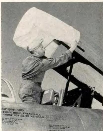
S/Sgt. Roy V. Matlock installs hood to prevent burning pressurization hose.
