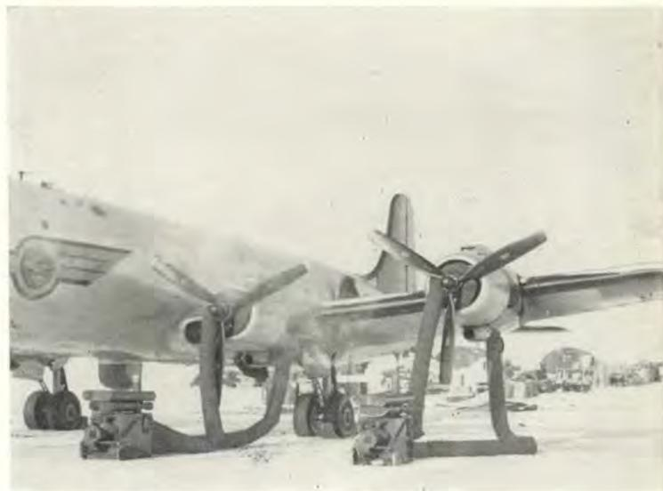
Engine heater hose can look like a bunch of overgrown snakes when multi-engine planes are being heated. Cockpit also gets heat.
