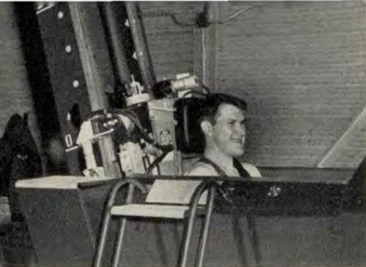
The ejection trainer operates out of a cockpit mockup and the seat is propelled from nine to 16 feet up the track.
