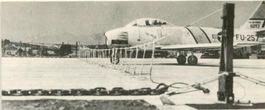
An F-86 moves down the runway and is shown prior to and immediately after initial contact with nylon webbing. Arresting cable will spring up to engage main gear.
