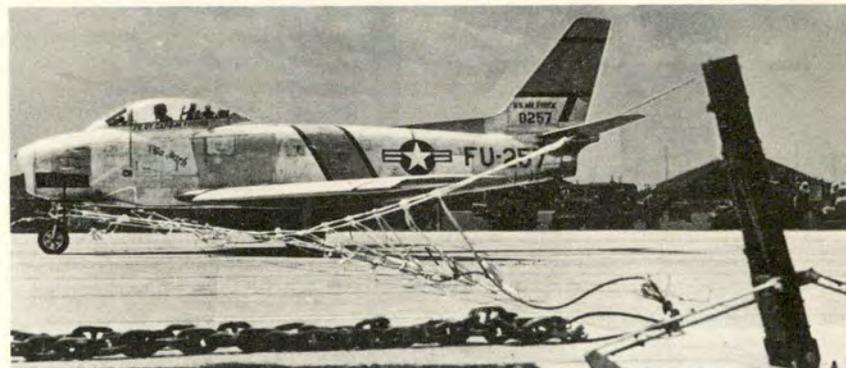
With the arresting cable now positioned and pulled taut, the aircraft begins to drag the heavy, linked chains which are stretched along both sides of the runway.
