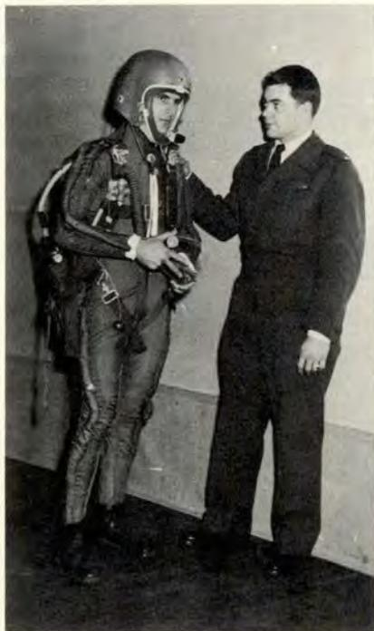
The XA-13, a semi-rigid helmet, designed primarily for the long-range bomber aircraft.
