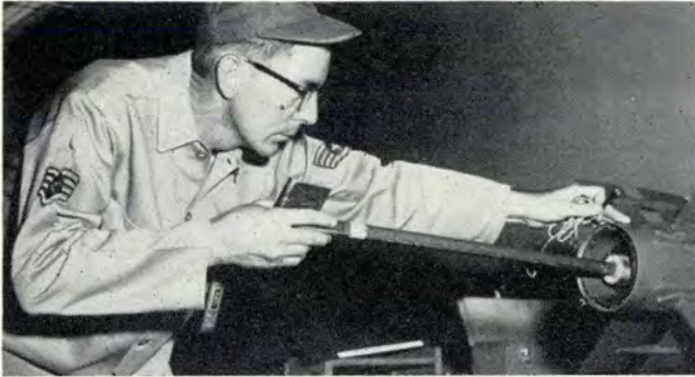
Above, Sgt Thomas removes the igniter from its container. Right, note the installation of a shorting clip across the pins of the igniter. This prevents accidental ignition from stray radio frequency energy. Below, Thomas inserts the igniter with a T-handle.
