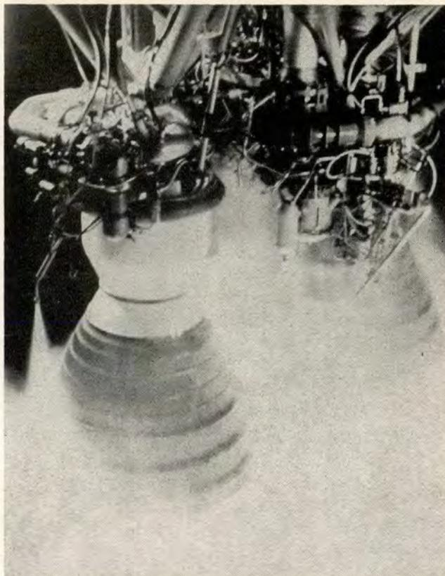
**Titan II first stage engine test firing. During SLAP approximately every third engine was static fired prior to teardown to test performance.**
