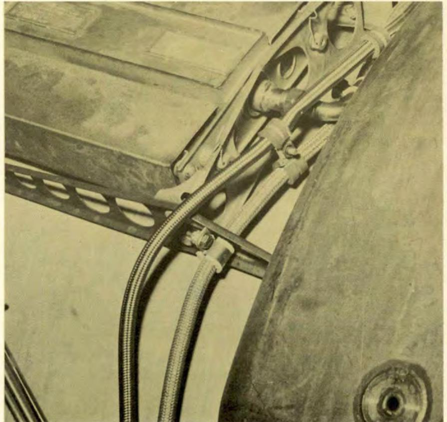
Conduit improperly clamped.
