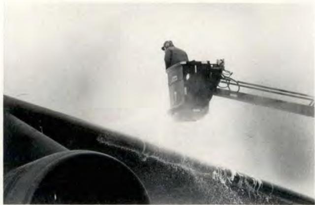
Deicing should be accomplished just prior to flight. Even short delays can result in further icing.
