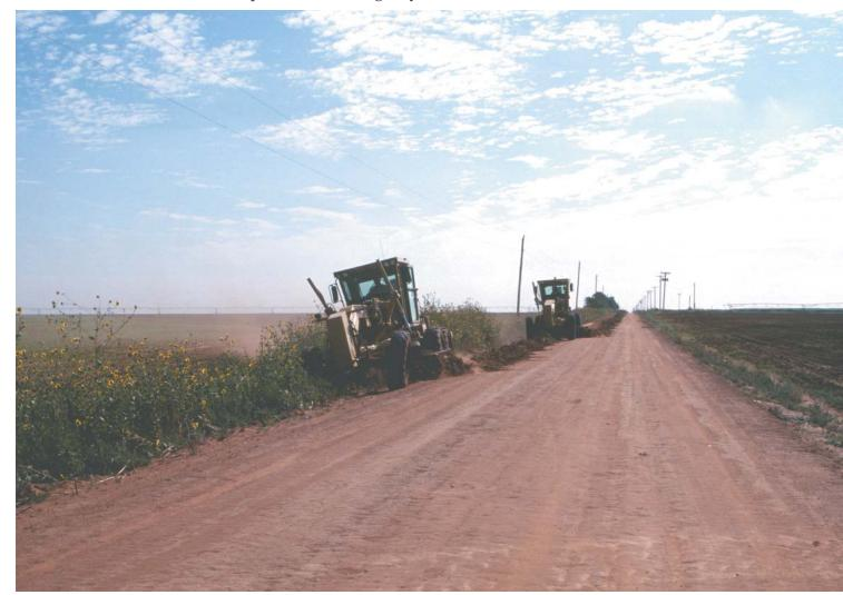
Curry County road maintenance personnel periodically grade the dirt road in an attempt to keep the surface drivable. However, frequent heavy rains and high winds during the summer and fall can cause heavy erosion, leaving a rutted, washboarded surface that can send a fast-moving vehicle out of control.
