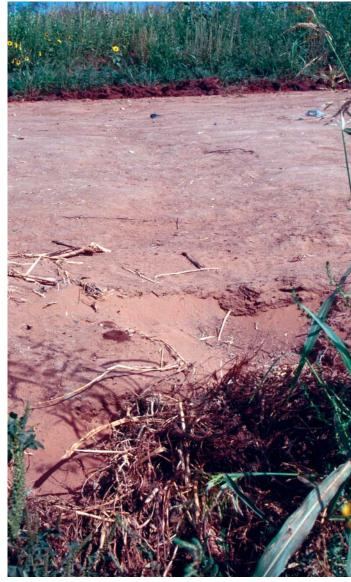
Dips in the road, even though periodically filled in by county maintenance, soon begin to erode as rains wash away the fill dirt. The errosion can be severe, creating dips deep enough to send a speeding vehicle out of control.
