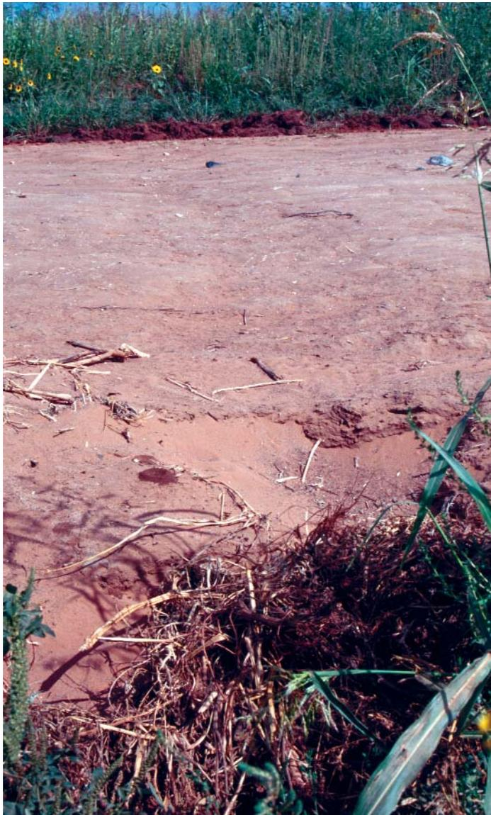
Dips in the road, even though periodically filled in by county maintenance, soon begin to erode as rains wash away the fill dirt. The erosion can be severe, creating dips deep enough to send a speeding vehicle out of control.
