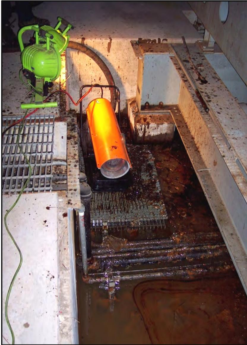
Figure E-1. Fluid Pumping from Pits.
